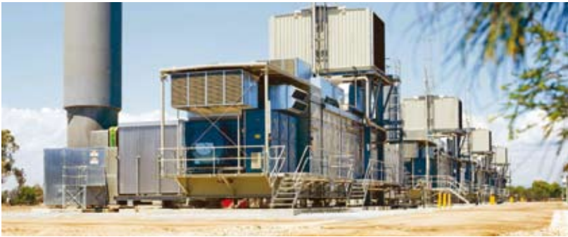
On Torrens Island, Australia, four SGT-600 gas turbines provide seasonal peaking support for the electrical grid.
