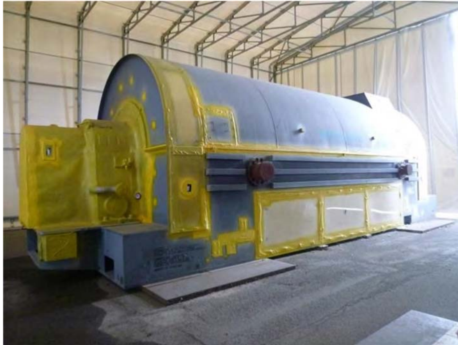
Figure 4: SIEMENS Generator SGen5-1000A
