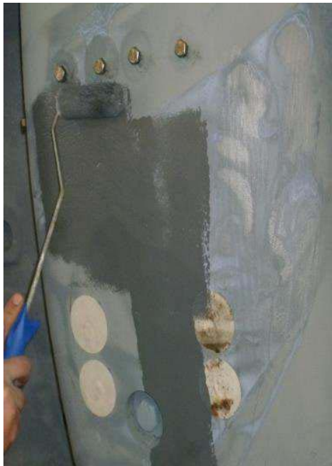
Figure 9 & 10: casing painting
