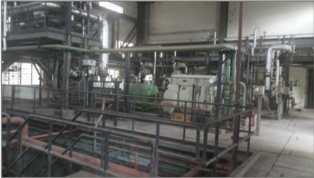
Condition of HP Boiler Feed Pumps
