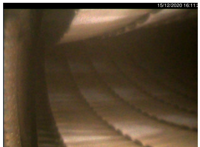
Picture 18: combustor outer liner
