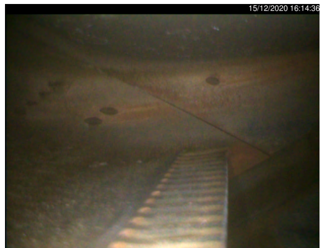
Picture 24: stage 1 nozzles, trailing edge
