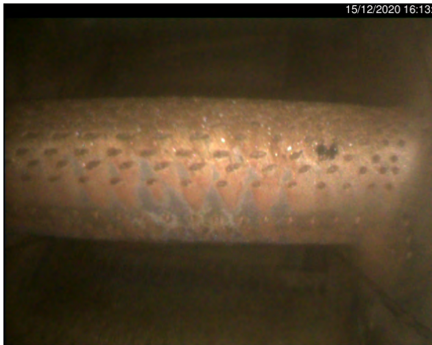
Picture 21: stage 1 nozzles, leading edge
