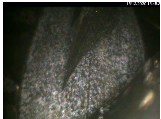
Picture 10: salts and deposits
