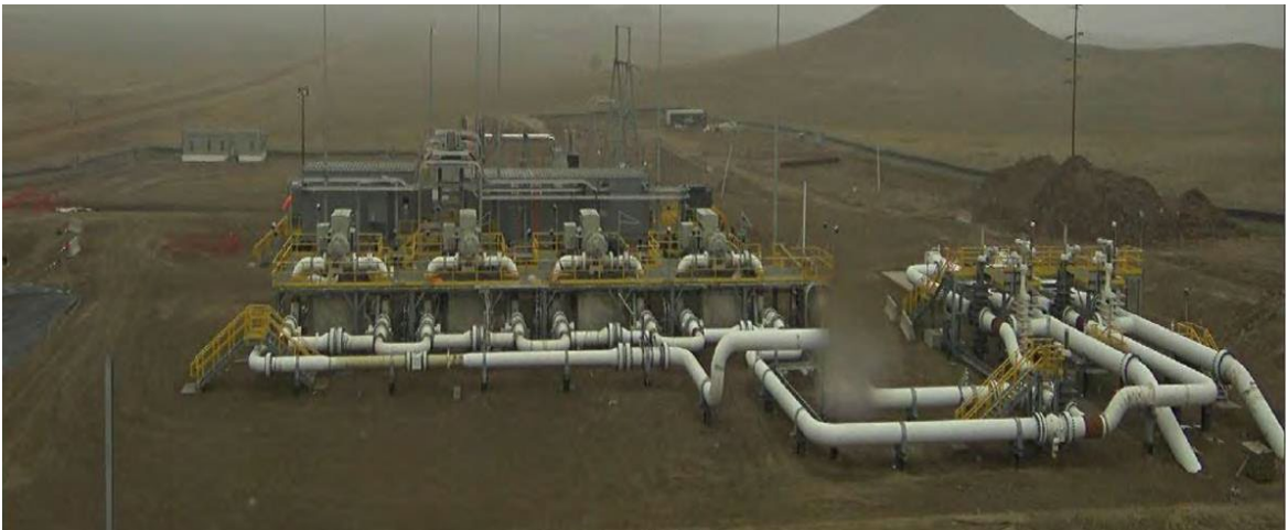
PUMP STATION 14 – 12 th April 2021
