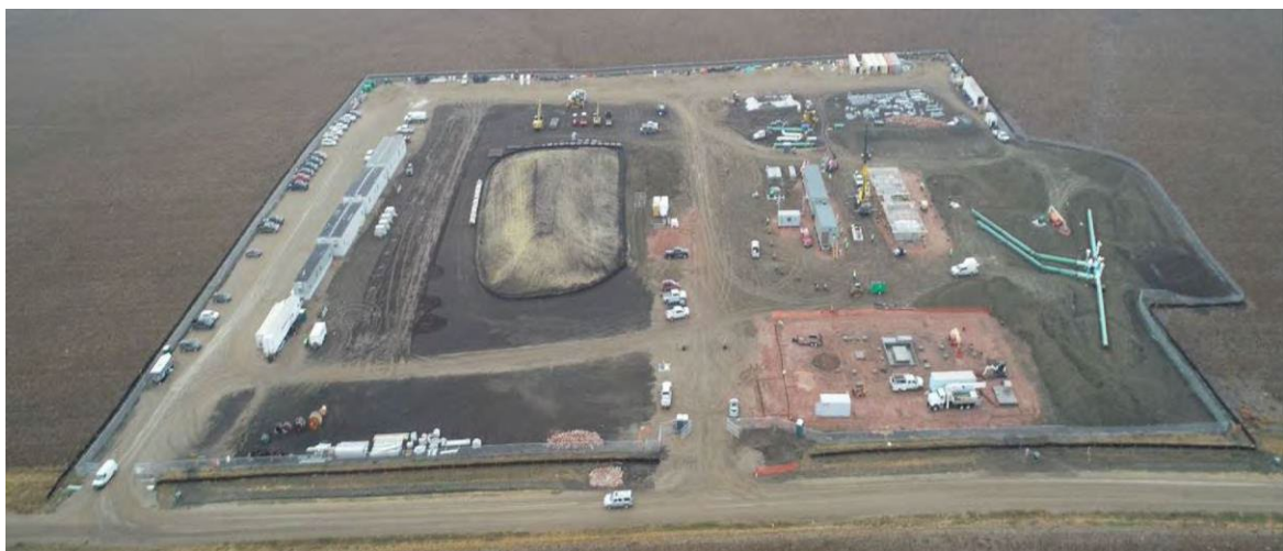
PUMP STATION 18 – October 2020
