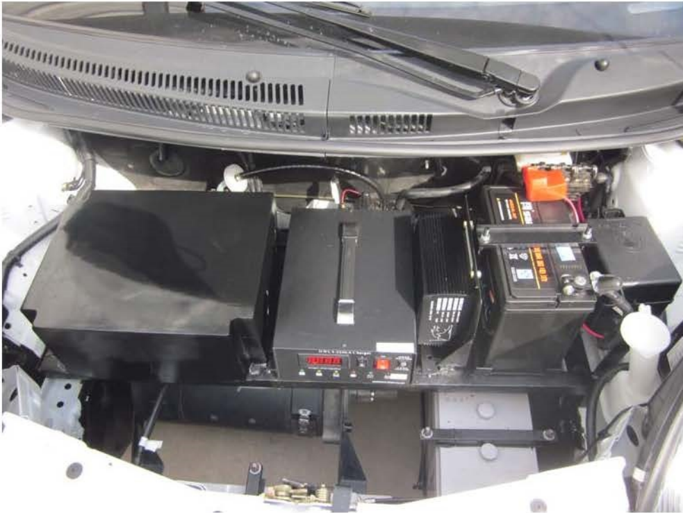
Electric Controller And Electric Motor
